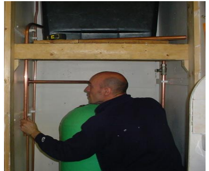
Installing an airing cupboard in copper
