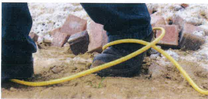
Cables can be a trip hazard on site
