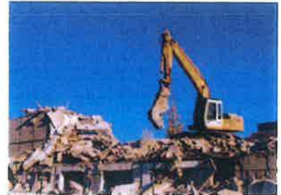
The CDM Regulations play a role in safety during demolition.
