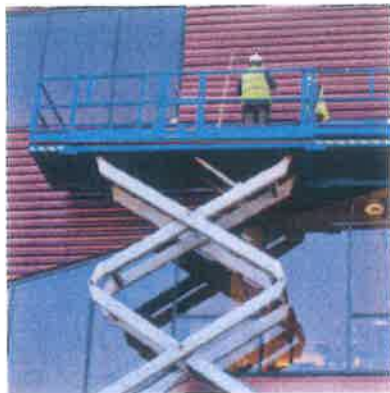
Using a scissor lift at height
