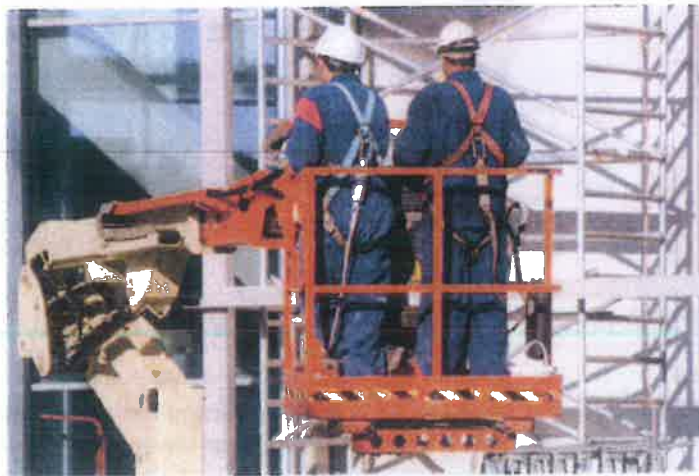
Workers wearing safety harnesses on an aerial access platform
