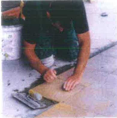
A tiler tiling a floor
