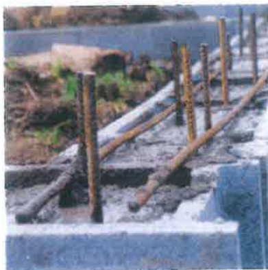
Concrete with steel reinforcement
