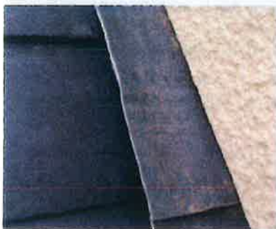
Flashing providing waterproofing
