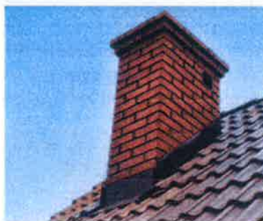
Flashing around a chimney
